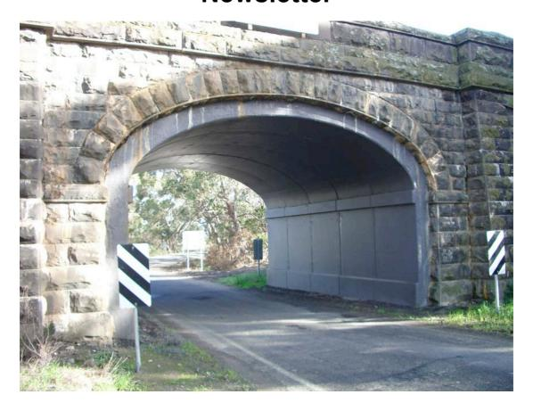
The Blue Bridge at Mount Doran, photographed in July 2009, showing the reinforcing works carried out by VicTrack in recent times, under the supervision of Heritage Victoria. The underside of the bluestone arch has been reinforced with steel, dramatically changing the appearance of the old bridge.
